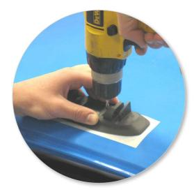
Drill through the two holes in the foot while holding foot tight on roof in marked position.
