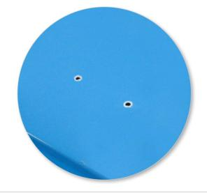
Remove masking tape and place silicon sealant around drilled holes on roof for all four positions.
